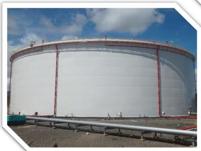
Floating Roof Tank of 95,000 m<sup>3</sup>
