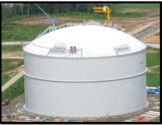
170,000 m³ Single-containment LNG Tank
