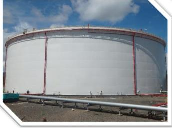
Floating Roof Tank of 95,000 m<sup>3</sup>
