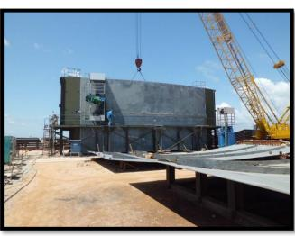
Shell Plate Pre-assembling at TKI Kabil Yard
