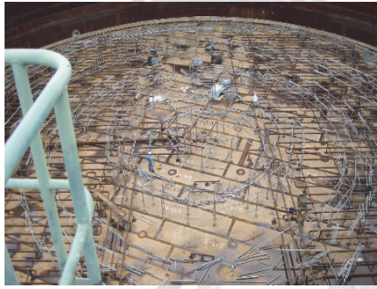
Construct New Floating Roof
