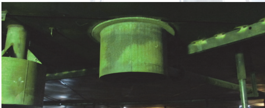
Floating Roof Drain System
