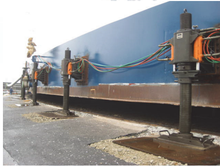
Lifting the Tank with Jacks
