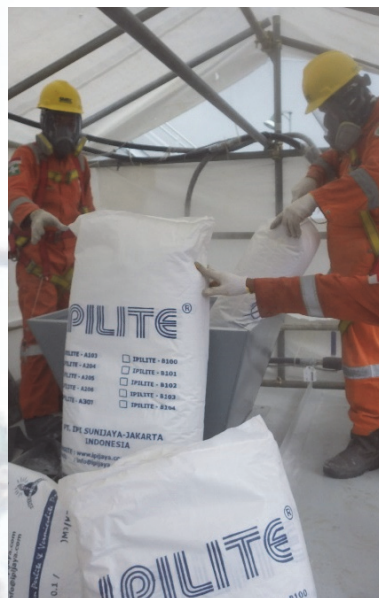
Perlite Hopper Installation for Topping-up
