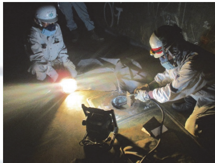
Patch Plate installation on the Bottom by lap weld
