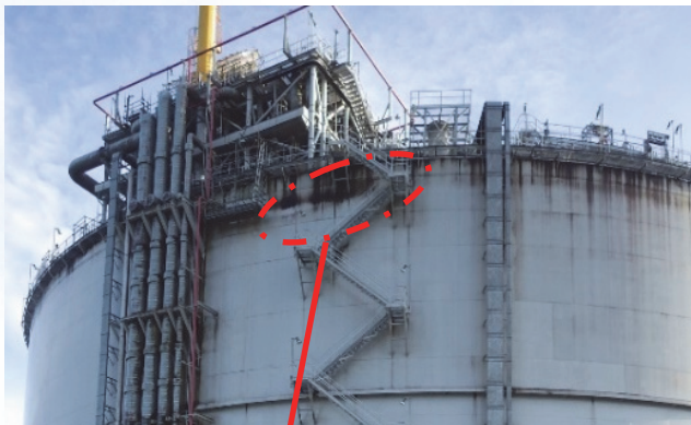
Frost on the shell plate monitored by Thermograph
