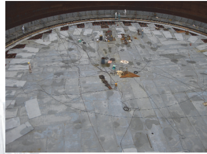
Construct New Floating Roof
