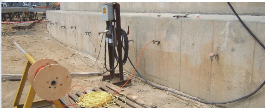
Bottom Heating System for Low Temperature Tank
