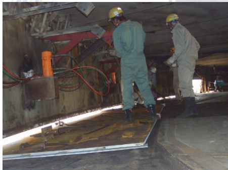
Annular and Bottom Plates Replacement
